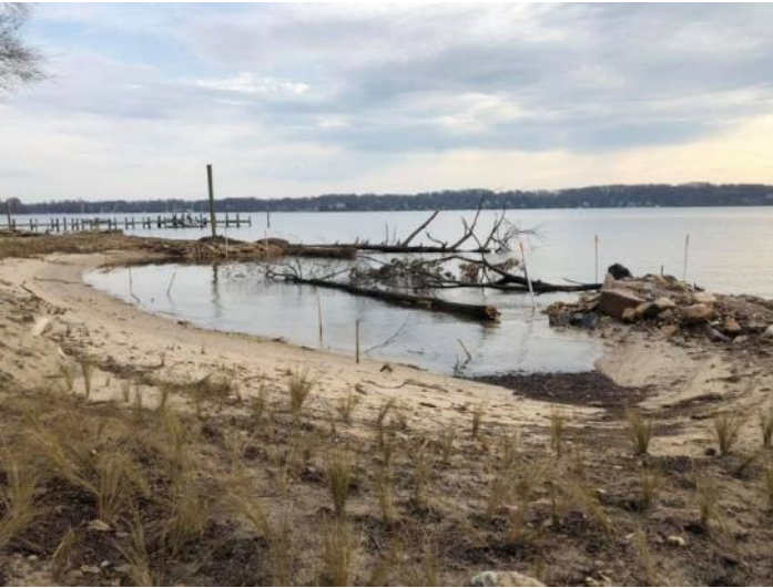
A living shoreline that was recently installed at Kyle Point on the Severn River. (Photo: Erik Michelsen)
