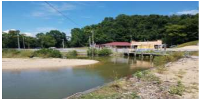
Existing Gilligan's Pier Restaurant at Pope's Creek
