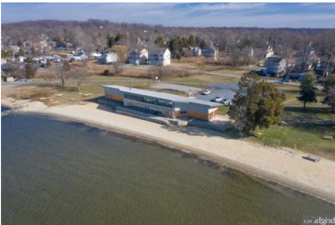
Selby Bay Community Beach Club House
