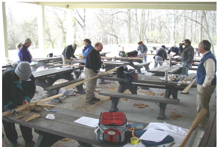
Cedar shavings turn Carderock pavilion into a giant gerbil cage Photo by Gina Cicotello
